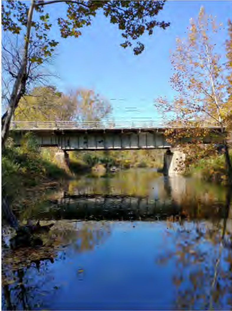
A bridge over the Normanskill on State Route 146 near Tawasentha Park. Bridges like this one may need to be re-engineered to properly accommodate cycling/pedestrian users as well as vehicles.
